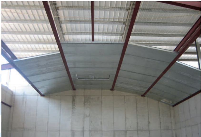
Hemi-anechoic chamber with a curved roof during construction phase
