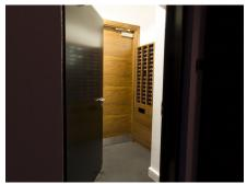
In addition to the Ray Dolby Lounge, the IAC doors were used to isolate smaller screening rooms, plus reduce the noise of the projection equipment to neighbouring offices.
