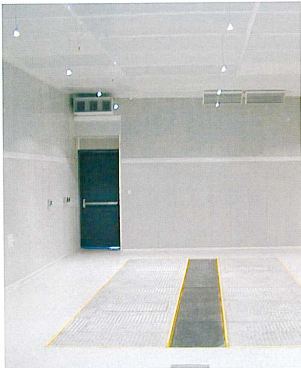
VIEW inside PlanarCHOIC Room designed and built for a world wide known car tyre manufacturer at point of carrying out the acoustic performance test.
