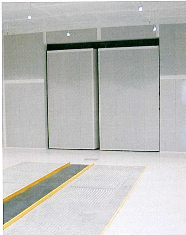
VIEW towards large acoustic entrance door inside PlanarCHOIC Room.
