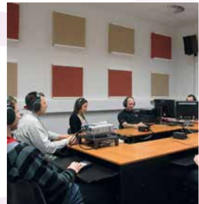
A typical IAC listening room installation
