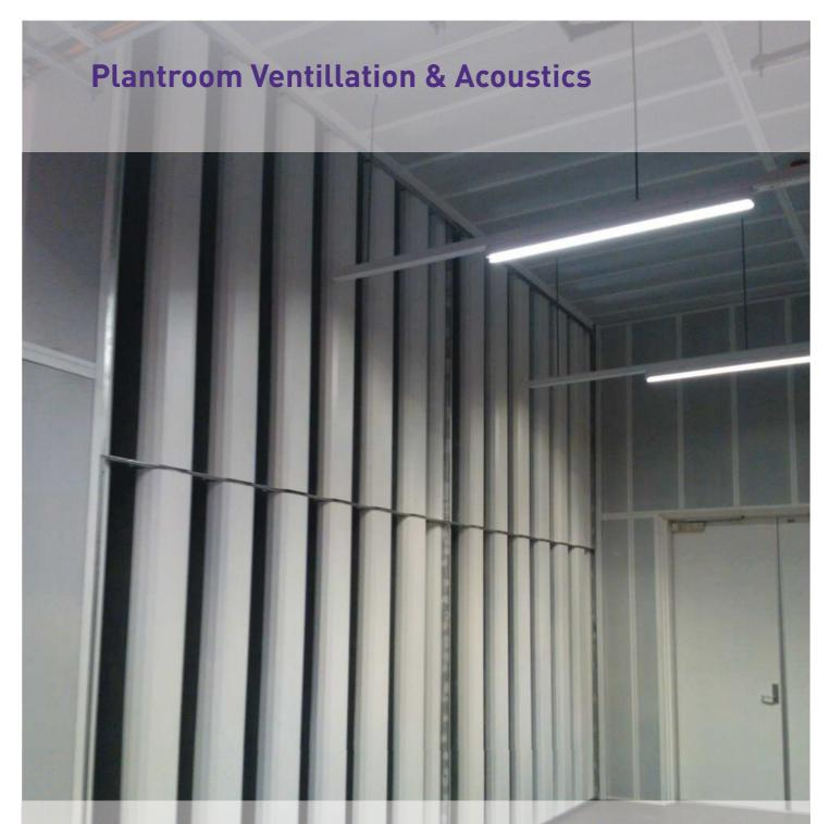
IAC Acoustics provide a complete solution to all ventilation requirements for enclosed diesel generator sets including attenuators, acoustic louvres, dampers, ducting and fans. These products serve the purpose of ensuring the correct level on ventilation is achieved, whilst minimising the effect of noise in areas adjacent to the plant room.
