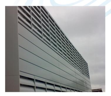
IAC designed, manufactured and installed a 50m long, 20m wide and 8m high acoustic compound to house generators at ground level and chillers on a mezzanine level. Backup power and cooling was transported into the building by means of an 18 tonne service gantry.
